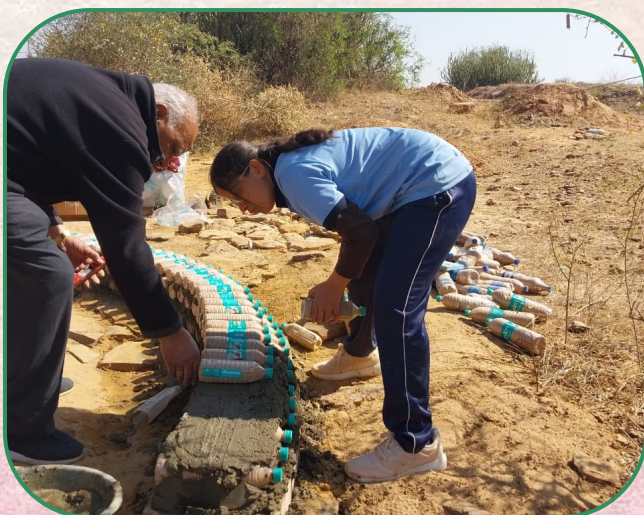
Eco Brick Otlā- Work in progress
