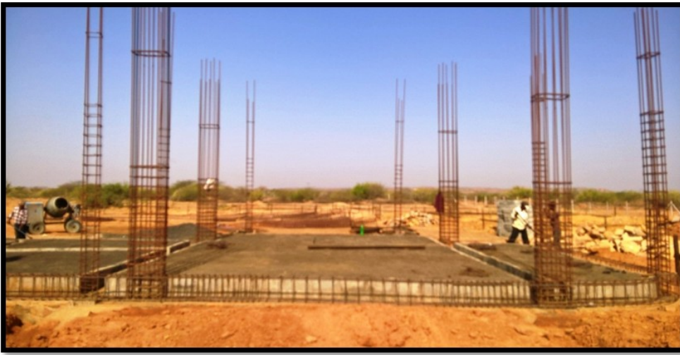
All ready for concrete base floor
