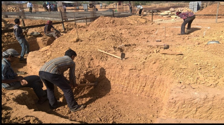
Digging foundations for columns
