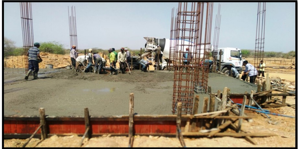
Working on base floor with ReadyMix Concrete
