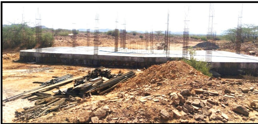
Base floors are ready for Block 2 and 3
